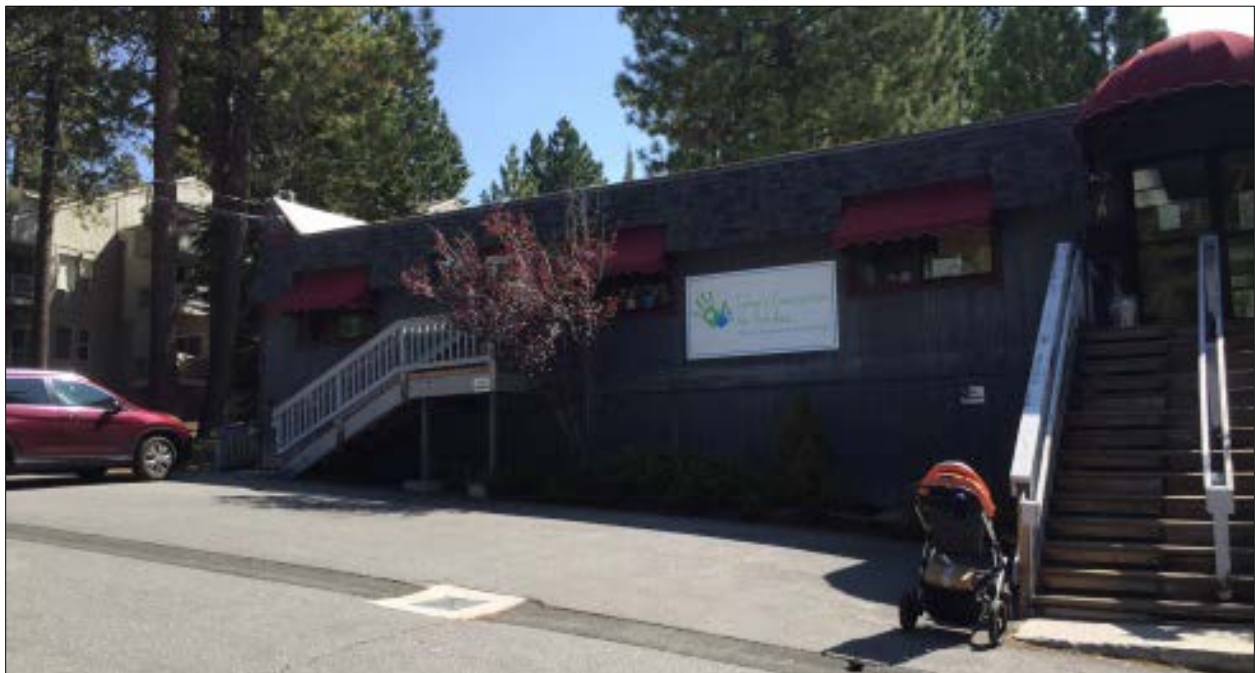
Entrance to building and front parking lot
