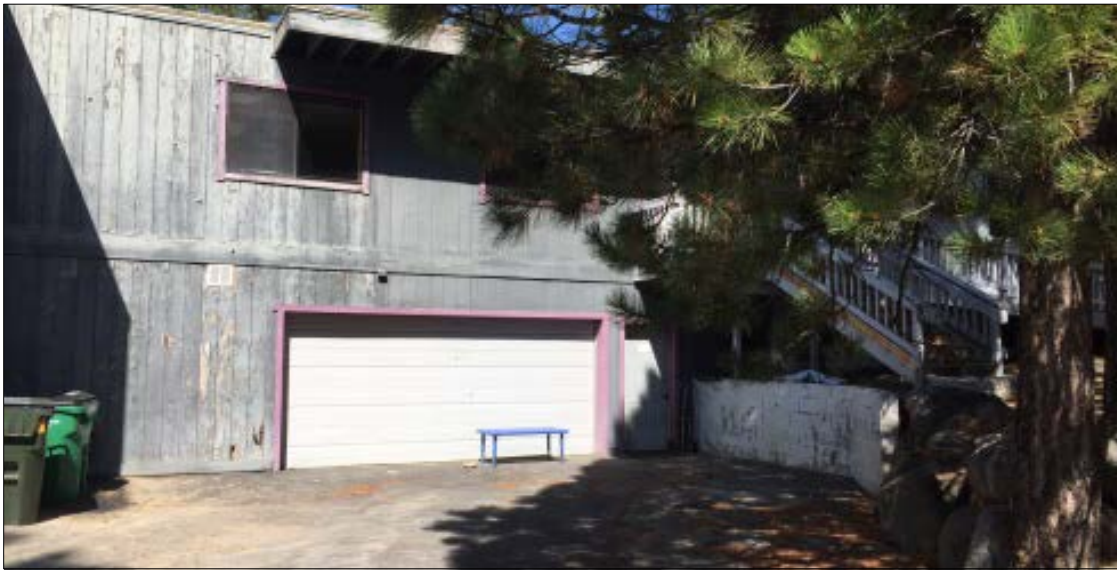
Rear of building – outside play area (to be fenced)
